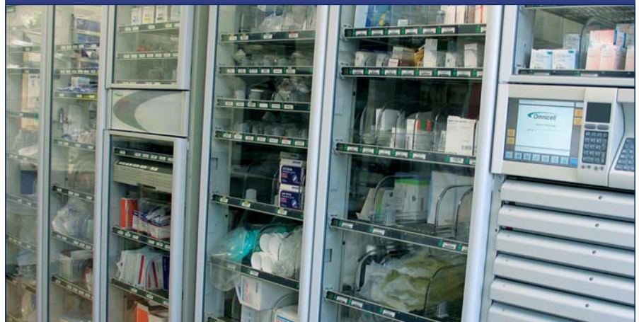
Figure 1: Main dispensing cabinet (pharmacy) with attached auxiliary cabinets (medical supplies) in the Department of Respiratory Medicine, Onze Lieve Vrouwe Gasthuis Hospital (Omnicell configuration)
